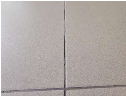
Foto 7: Rejected joint.
