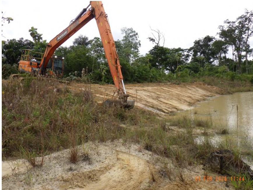
Figure 9.3 Reprofiling the open-mining pit to ensure slope stability and safer access
