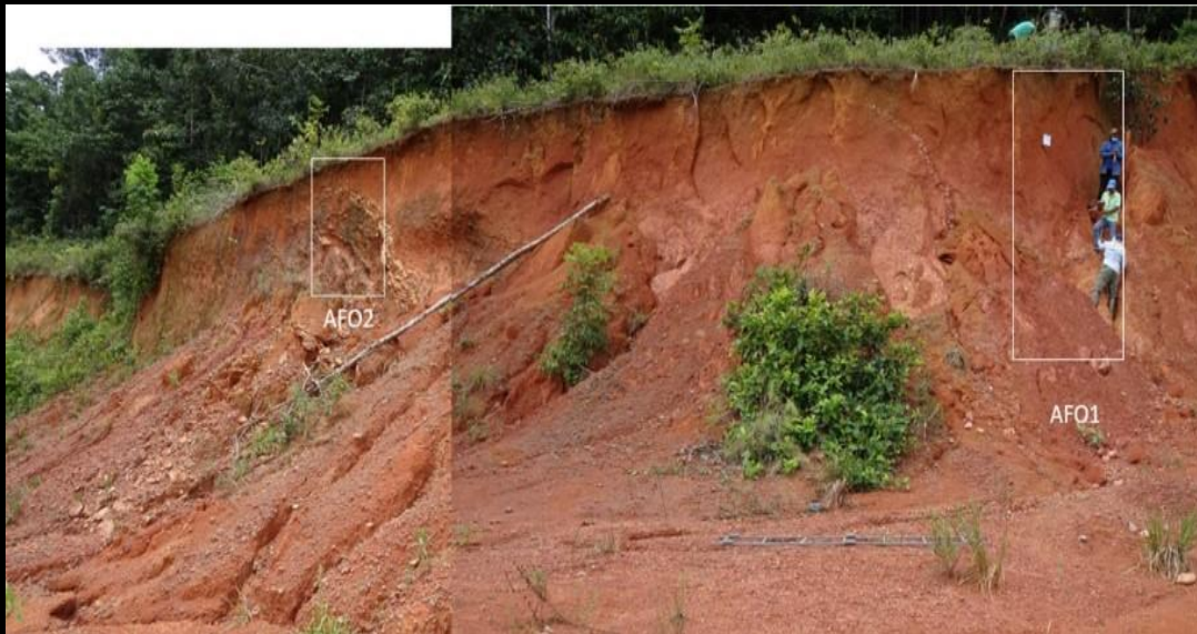
Panorama pilot site Afobaka Road km 55, 2021
