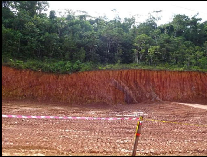
Test site Afobaka Road km 55, 2017: anticlinal fold structure in Paramaka rocks
